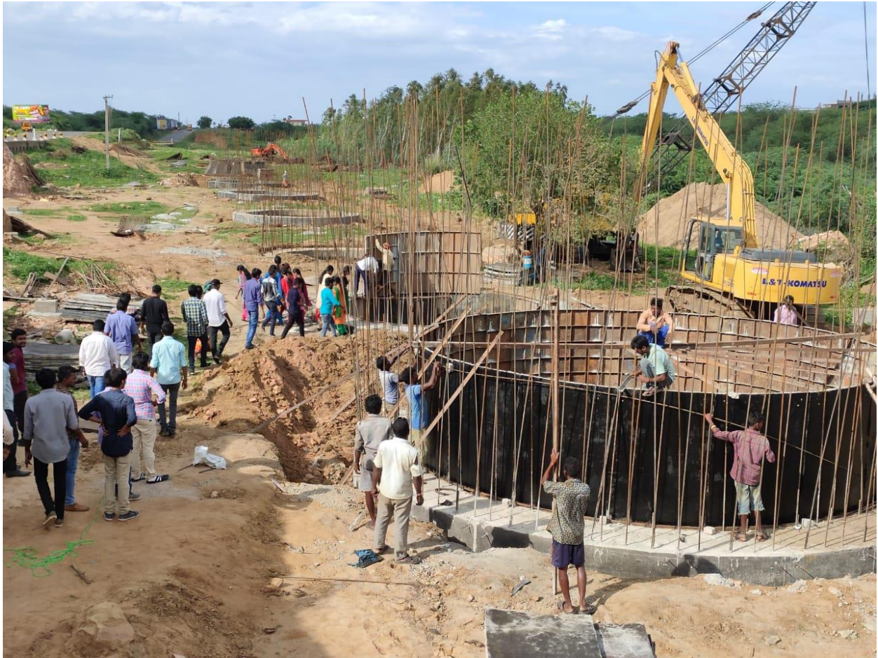
Students observing various components of Bridge.
